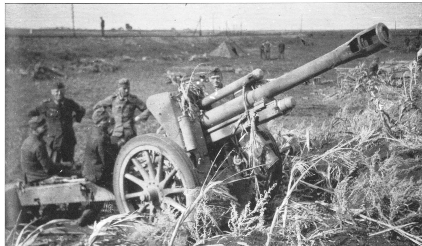
Two photographs showing gun crews preparing to fire modified 10.5cm le FH 18/42 guns in anger. The 10.5cm was the standard light artillery piece deployed in the artillery divisions on the Eastern Front. However, in order to give the gun better punch on the battlefield the weapon was modified in 1942. The barrel was lengthened, a cage muzzle-brake was fitted, and the carriage was a lightened version of the le FH 18 design.
