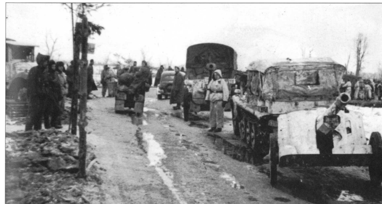
A column of vehicles have halted on an icy road on the Narva Front in February 1944. A whitewashed 7.5cm Pak 97/38 and a captured Russian 7.62cm Pak anti-tank gun can be seen on tow. Note the Kettenkrad passing the stationary vehicles. This tough little tracked vehicle was powered by an Opel Olympia gasoline engine, which developed 37 hp at 3400 rpm.
