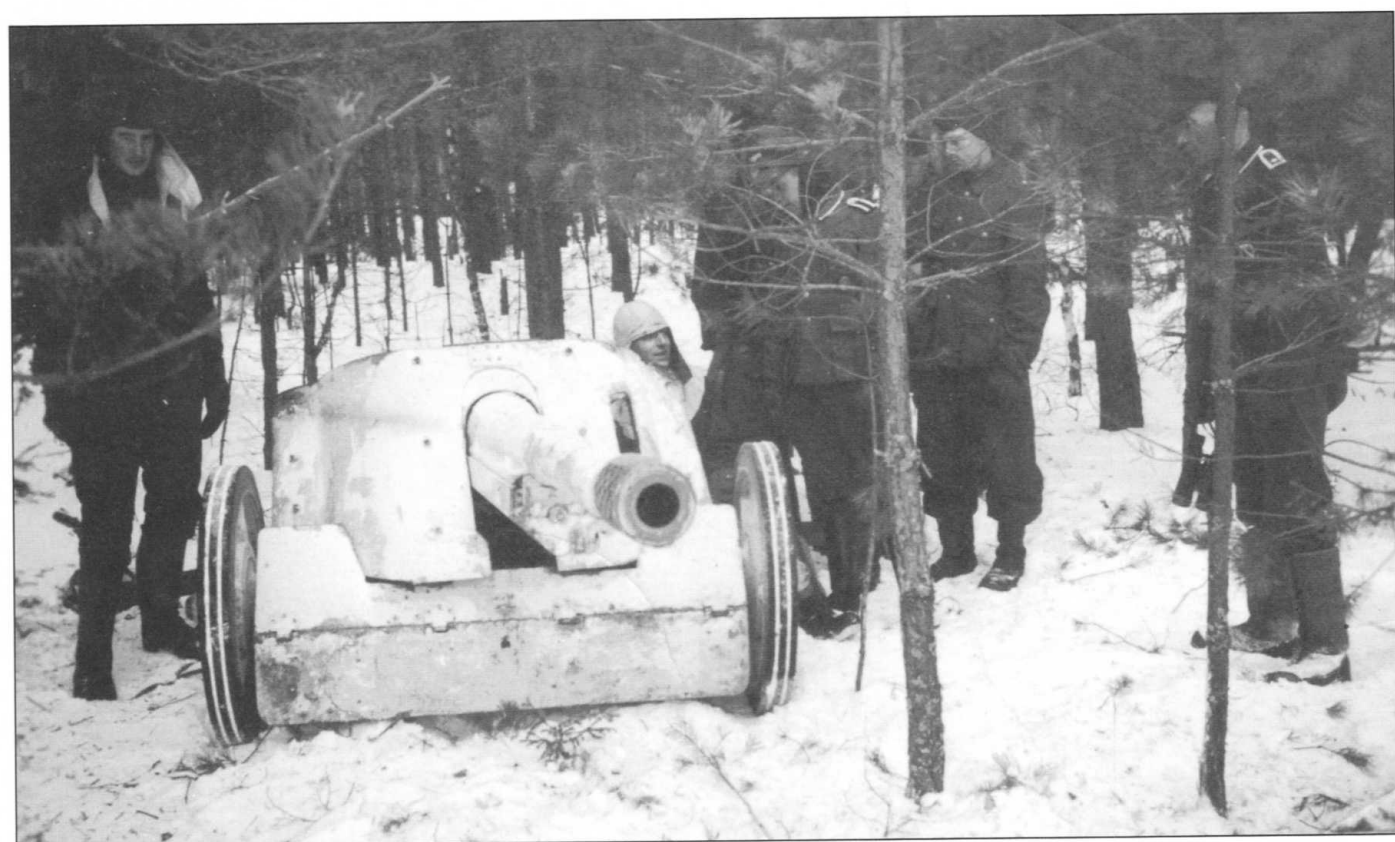
Well concealed inside a wooded area the crew of white-washed 7.5cm Pak40 can be seen with their deadly anti-tank weapon. The Pak40 had spaced-armour shield which was held together by large bolts. These bolts also had drilled holes that allowed the crews to thread foliage through them.
