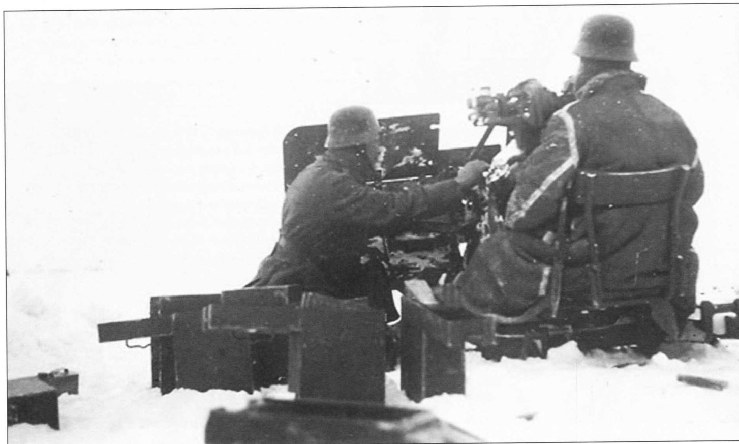
Out in the snow and the crew of a 2cm Flak gun are in action. The gun was a very effective weapon and had a fire rate of 120-280 rounds per minute. The weapon's rate of fire was more than capable of dealing with attacking enemy troop concentrations. Note the amount of expended ammunition cases that are lying around the position.
