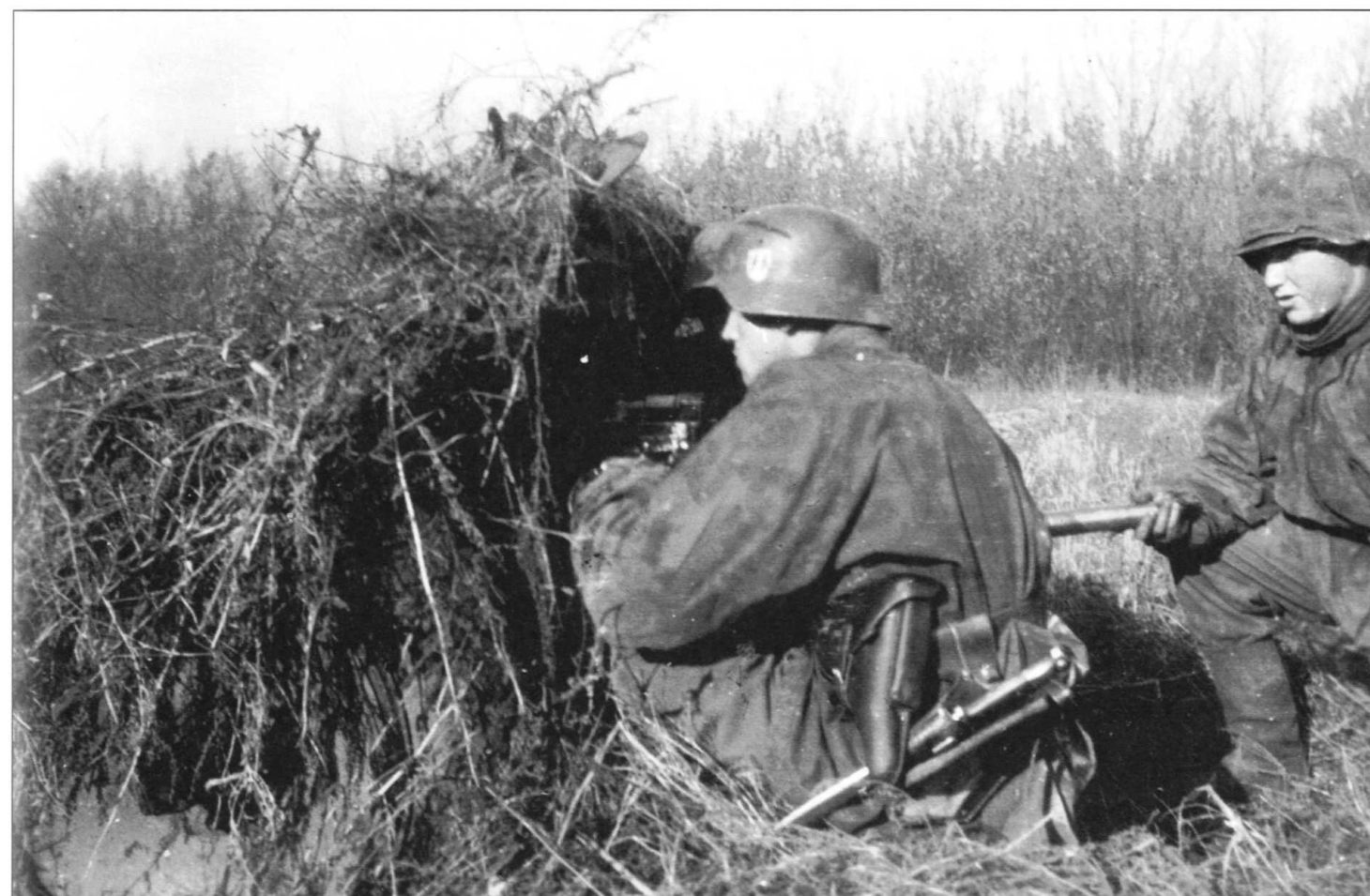
A well-concealed Waffen-SS Pak 35/36. The Pak 35/36 was the first anti-tank weapon to serve both the Wehrmacht and Waffen-SS. However, by the time it saw its debut on the Eastern Front the German gunners soon realized how limited the weapon was in an anti-tank capability. In spite of its inadequate fire capability the weapon still saw extensive action during the last years of the war including many defensive actions in the Baltics.
